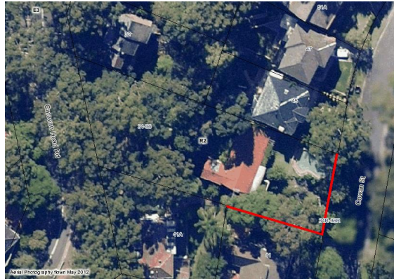
Aerial View: 34-36 Caravan Head Road- subject land (34R-36R) in red
